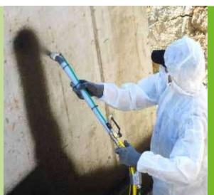
The **inoBEAM M8** delivery pump handles materials based on the "walk principle". A flexible rubber disc pushes the material to be conveyed through the pump housing and into the material hose.
